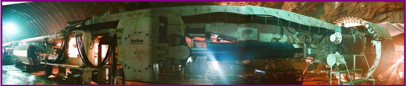
TBM Setup in Po Shan Tunnel
