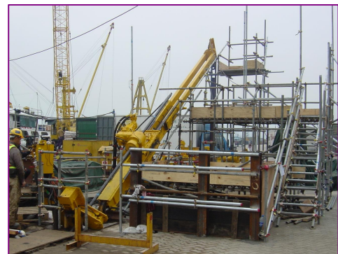
Setup of HD04 at Western Cargo Handling Area
